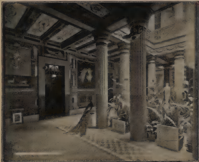
PERISTYLE OF THE POMPEIIAN HOUSE AT SARATOGA SPRINGS, N. Y. Franklin W. Smith, architect.
